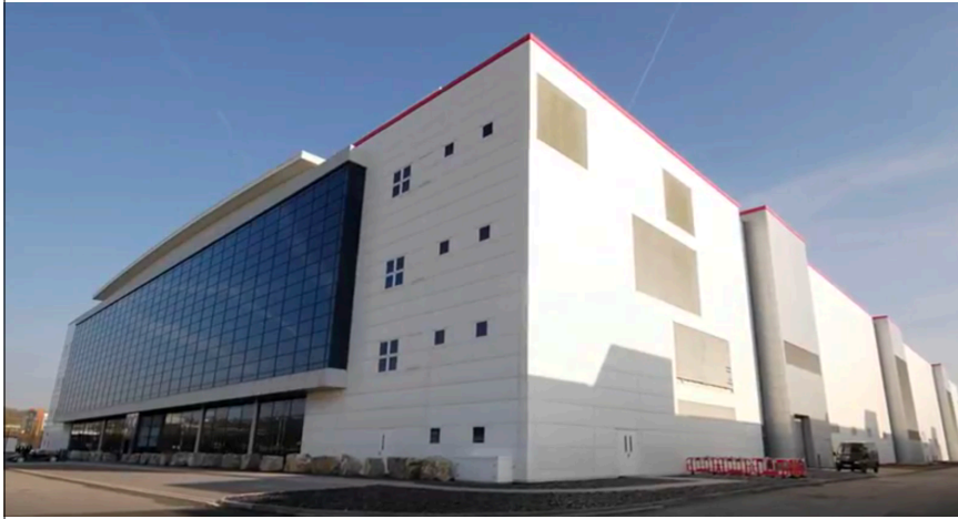
Platz 9: Next Generation Data Europe , Wales UK, Europe's largest Data Centre for powerful cloud services, with 22000 racks over a million square feet.
