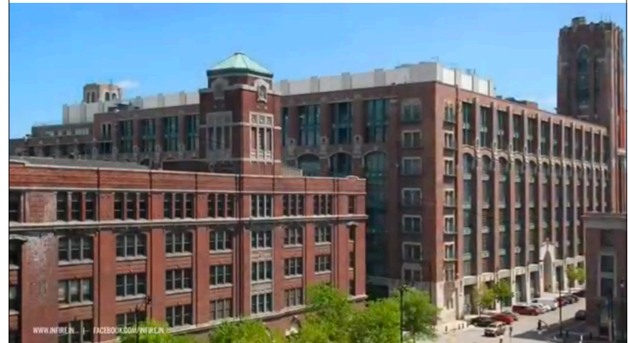
Platz 6: Lakeside Technology Centre , Chicago USA, 1,1 Mio Sq.Ft., building with more than 100 megawatts of power (Facebook, IBM...).
