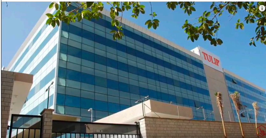
Platz 7: Tulip Data Center , Bangalore India, 1 Mio Sq. Ft., largest data centre outside US and largest in Asia.
